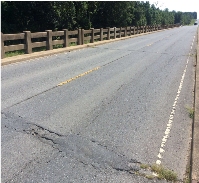
PHOTO 4 Description Wearing surface - Span 2 (cracking)
