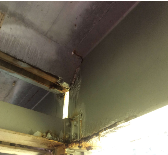
PHOTO 4 Description Span 10 Girder 1 @ Bent 10 (corrosion)
