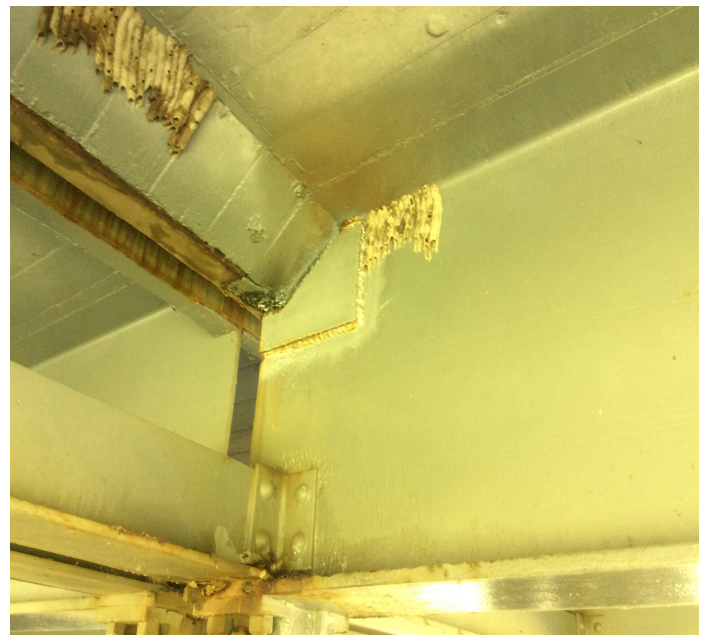
PHOTO 2 Description Span 2 Girder 3 right @ Bent 2 (corrosion)
