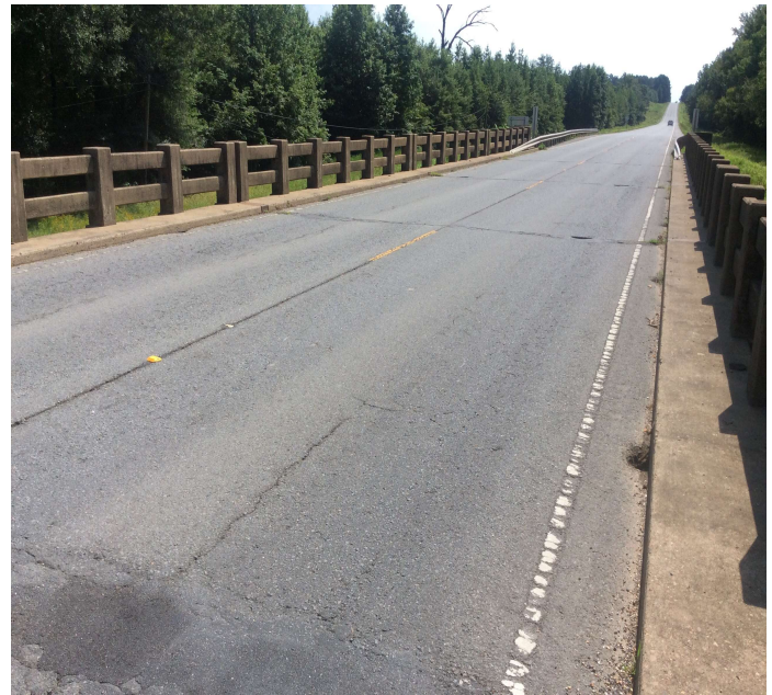
PHOTO 2 Description Wearing surface - Spans 8-10 right (cracking)
