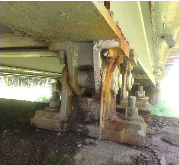
PHOTO 4 Description Bent 6 Bearing 1 ahead (corrosion)
