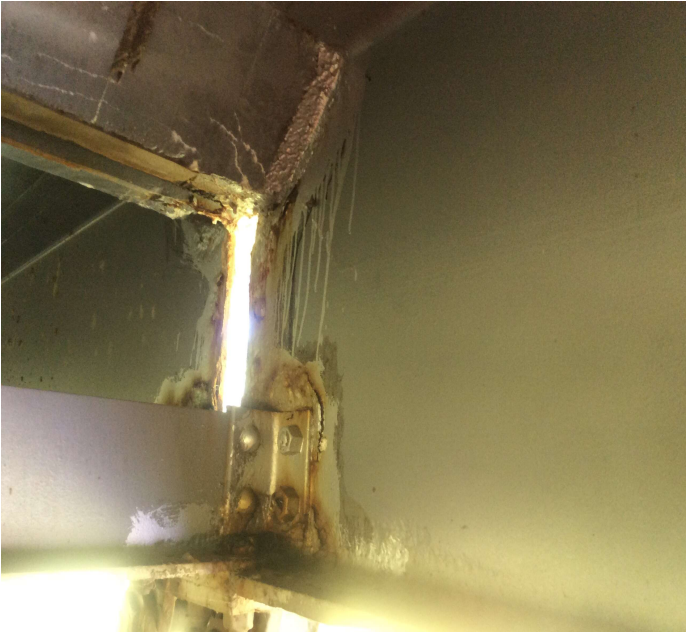
PHOTO 3 Description Span 6 Girder 1 right @ Bent 6 (corrosion)
