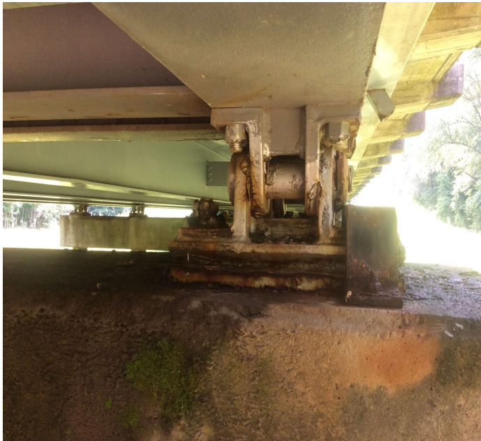
PHOTO 1 Description Bent 9 Bearing 5 back (corrosion)
