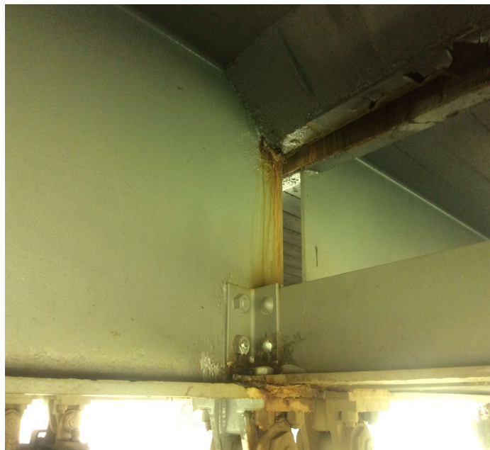
PHOTO 1 Description Span 5 Girder 3 left @ Bent 5 (corrosion)
