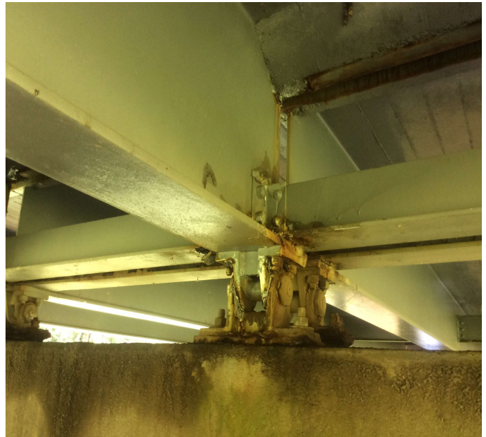
PHOTO 2 Description Bent 10 Bearing 3 ahead (corrosion)
