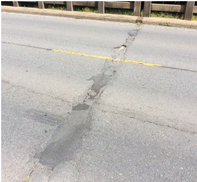
PHOTO 1 Description Wearing surface - Bent 11 (spalling)
