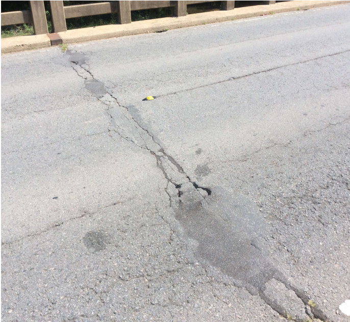
PHOTO 3 Description Wearing surface - Bent 6 (patches)
