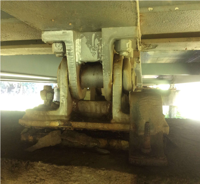
PHOTO 3 Description Bent 5 Bearing 4 back (corrosion)
